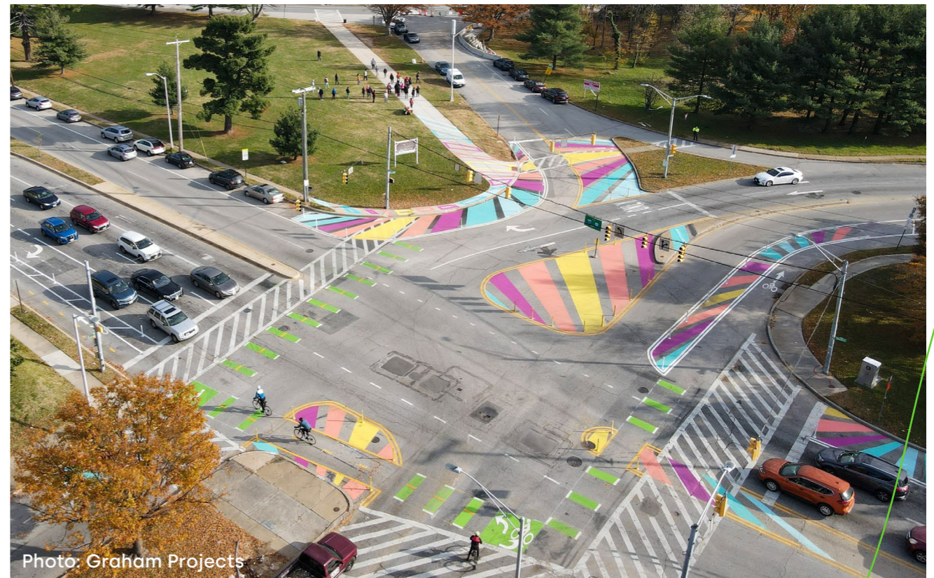
The new gateway to Lake Montebello Park slows vehicle speeds and improves safety for cyclists and pedestrians.
