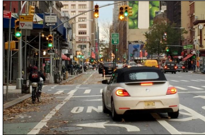
Split LPI w/ bicycle signal: 8th Avenue & W 29th Street, 2015
