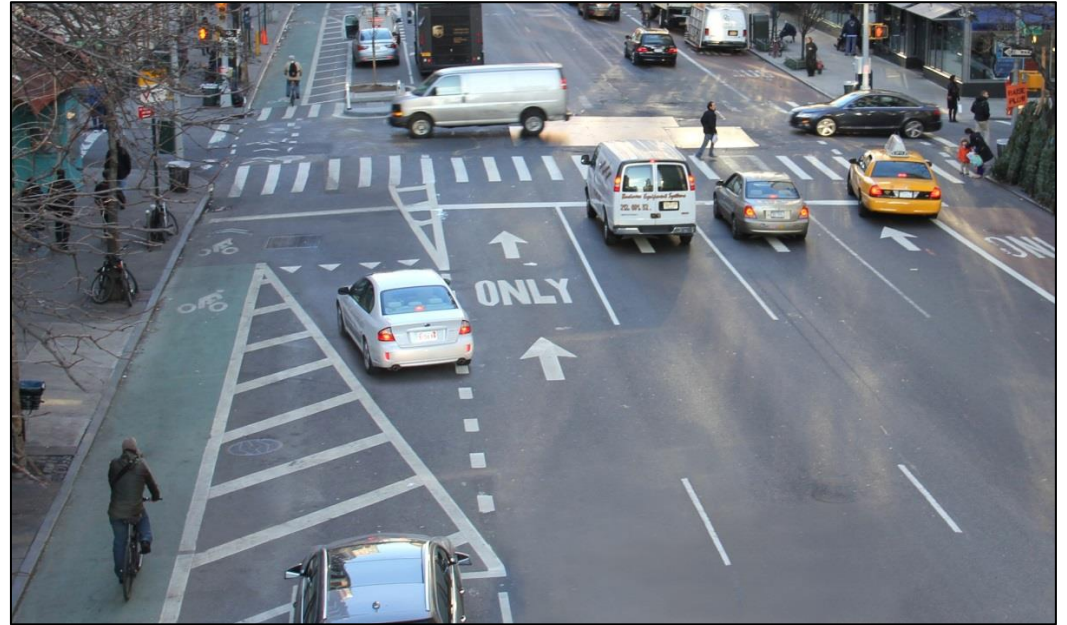
Protected bicycle lane on 1 st Avenue in Manhattan
