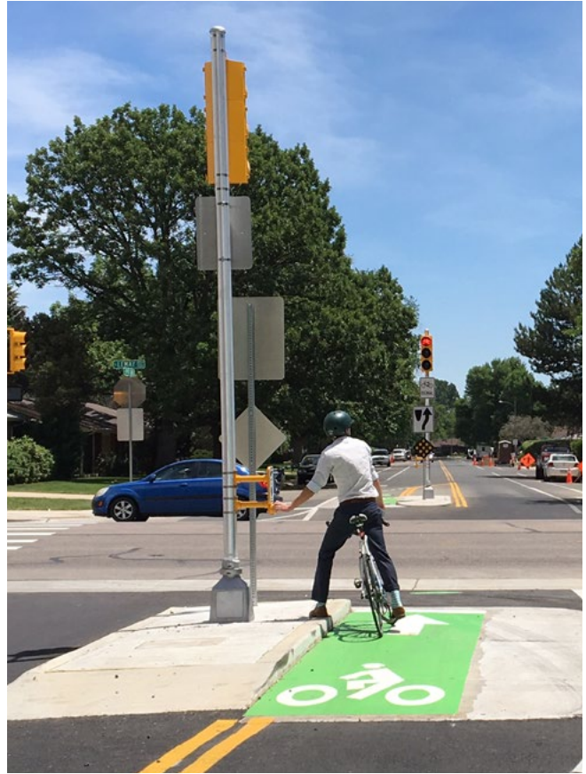
This push button has been extended to make it more accessible (credit: City of Fort Collins)
