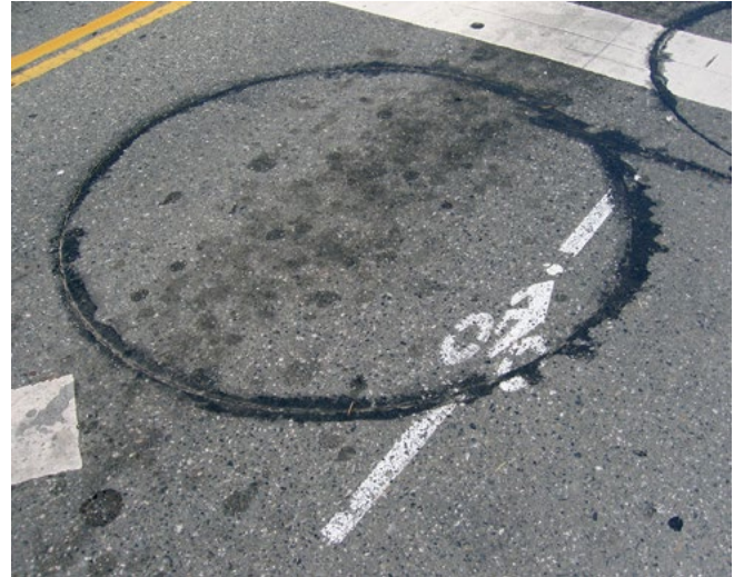
This 2009 edition MUTCD pavement detector marking is indicating to bicyclists where to wait in this shared lane so that they are on the most sensitive part of the Type E circular loop detector.
