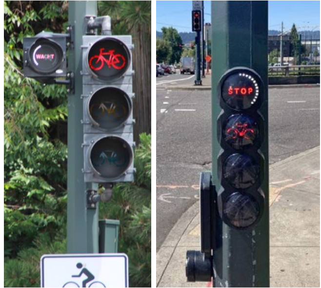
2015 Bicycle signal countdown timer (left) accompanies bicycle signal and activates upon detection of bicyclists. WACHT message modified to display WAIT. Nearside countdown timer (right) installed in 2020.
