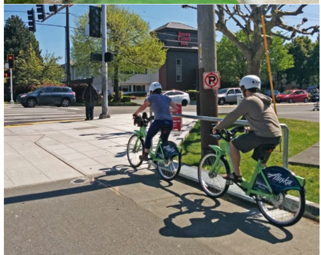
Bicycle lean rails installed within separated bike lanes in Charlotte, NC (top) and Seattle, WA (bottom)
