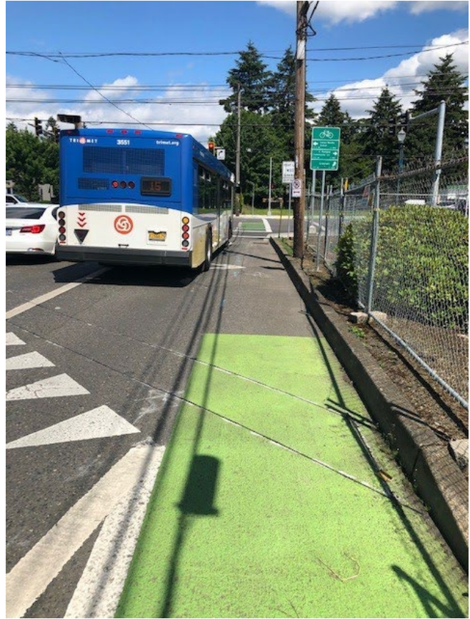
Parallelogram Loop Detector Configuration in Portland, Oregon detects bicyclists and vehicles entering this mixing zone. This location puts in a locking call and extended green for bicyclists. (Credit: Oliver Smith)
