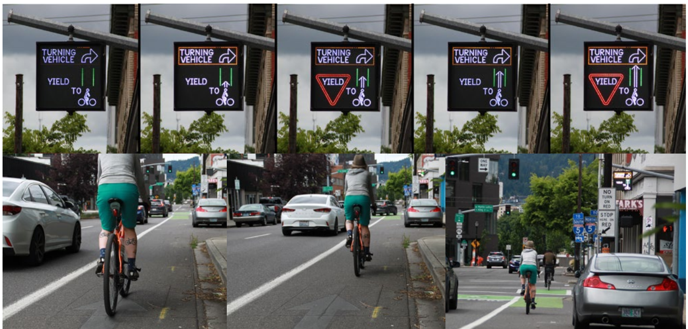
Above: LED sign sequence. Below: Left to Right: 1) Bicyclist rolls onto advance detector during green phase. 2) Blank-out sign (upper right of image) actuates. 3) Close-up of right-turning driver yielding to bicyclist while blank-out sign is displayed.
