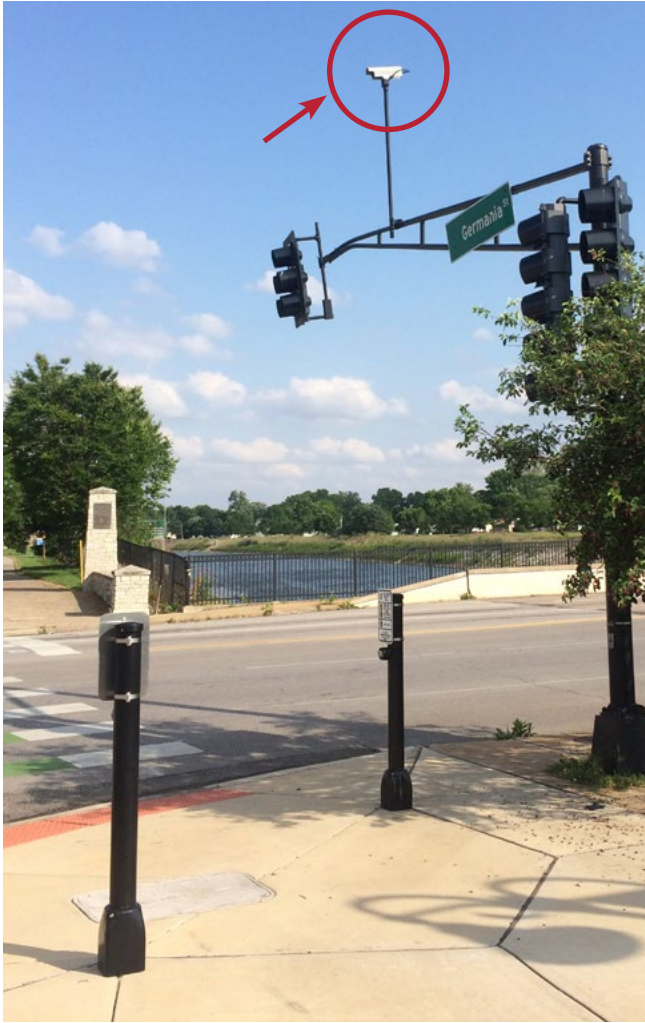
This camera in Missouri has been raised in elevation to obtain a better view of the intersection and its detection zones
