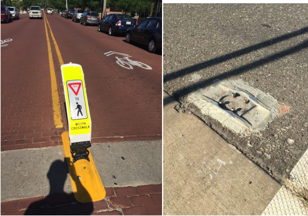
Figure 7.2. Figure 7.2a (above left) shows an R1-6 sign installed on a removable curb base that was damaged during the study. Figure 7.2b (above right) shows a sheared base of a flush mounted sign.
