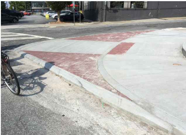
Pavers with concrete to denote walking path (Atlanta, GA)
