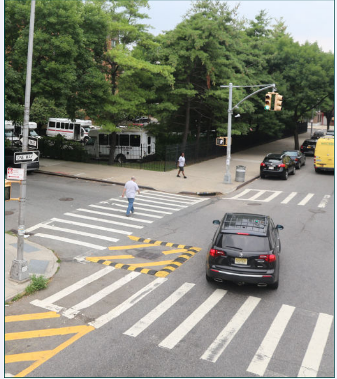
ABOVE LEFT: a passenger vehicle turns left at the intersection of two one-way streets, steering around a rounded corner apron with diagonal speed humps. Credit: NYC DOT. ABOVE RIGHT: an example of a square corner apron outlined with speed bumps. Credit: NYC DOT.
