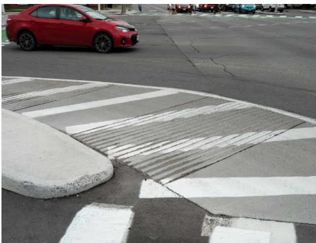
Flush with roadway (Ottawa, ON)
