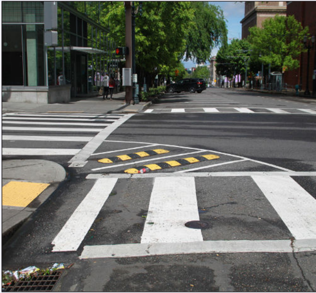
ABOVE LEFT: A corner “wedge” at the intersection of two one-way streets in downtown Portland. ABOVE RIGHT: A concrete corner speed hump as a right turn treatment. Part of the center area of the apron is raised as a deterrent to passenger vehicles. BELOW: A second example of a concrete corner speed hump, with a more pronounced “hump” area.
