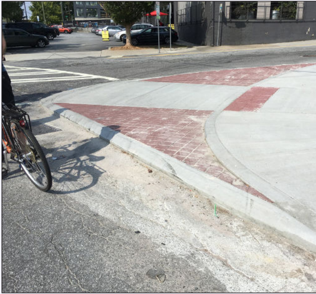
ABOVE LEFT: The corner design treatment applied at 10th NW and Brady. The apron is defined by a mountable curb with a significant vertical component. ABOVE RIGHT: The corner design at Peachtree Center and John Portman. BELOW: Two bicyclists queuing behind the mountable corner apron at Peachtree Center and John Portman.
