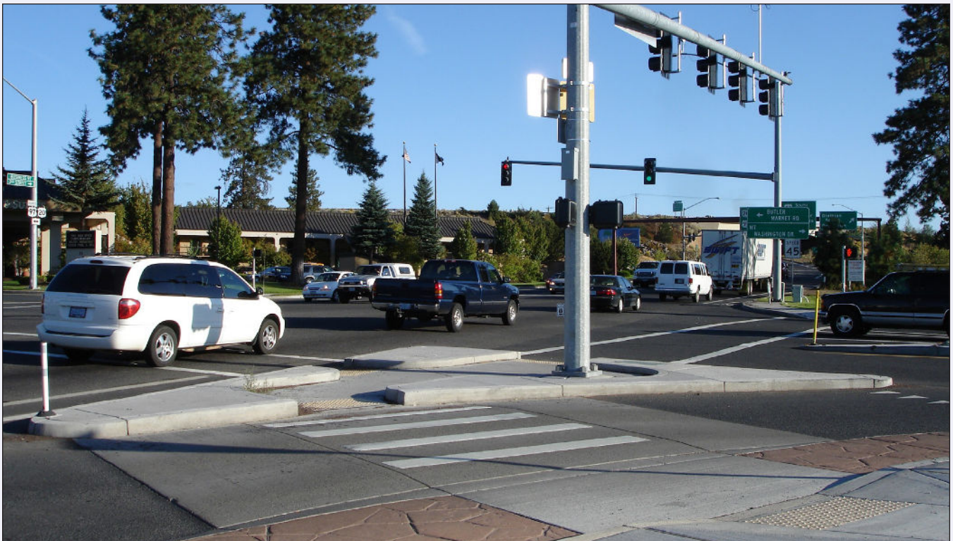
BELOW: A pedestrian's view of the channel crossing, showing the raised crosswalk and dropped curb.
