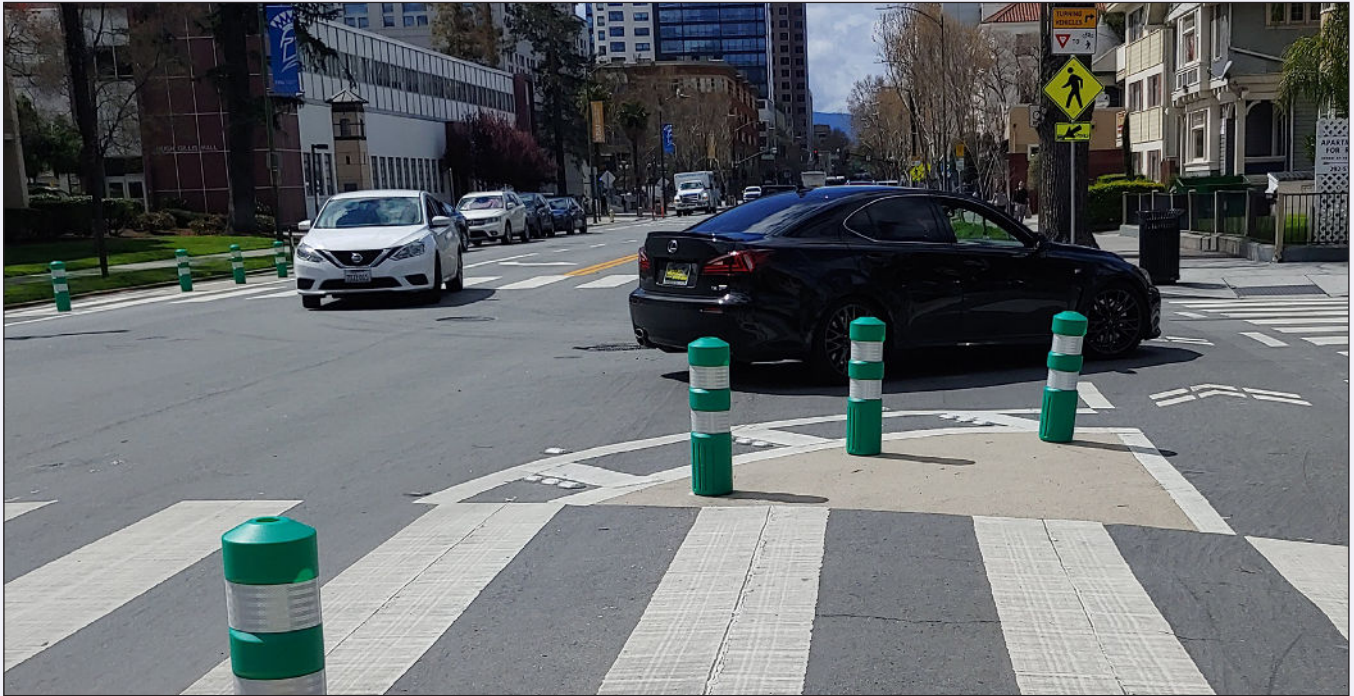
One corner of a quick-build protected intersection. A dual turning path is provided, and a passenger car is seen taking the managed vehicle path (smaller radius). Credit: City of San José, Department of Transportation
