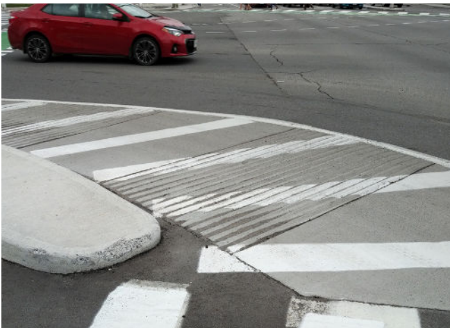
Rumble strips/surface (Ottawa, ON)
