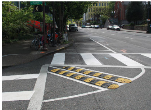
Speed bumps, defined turning path (Portland, OR)
