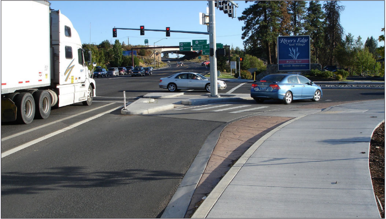
ABOVE: A view of the approach to the right turn channel showing the raised apron surfaced with stamped concrete and lined with a mountable curb.
