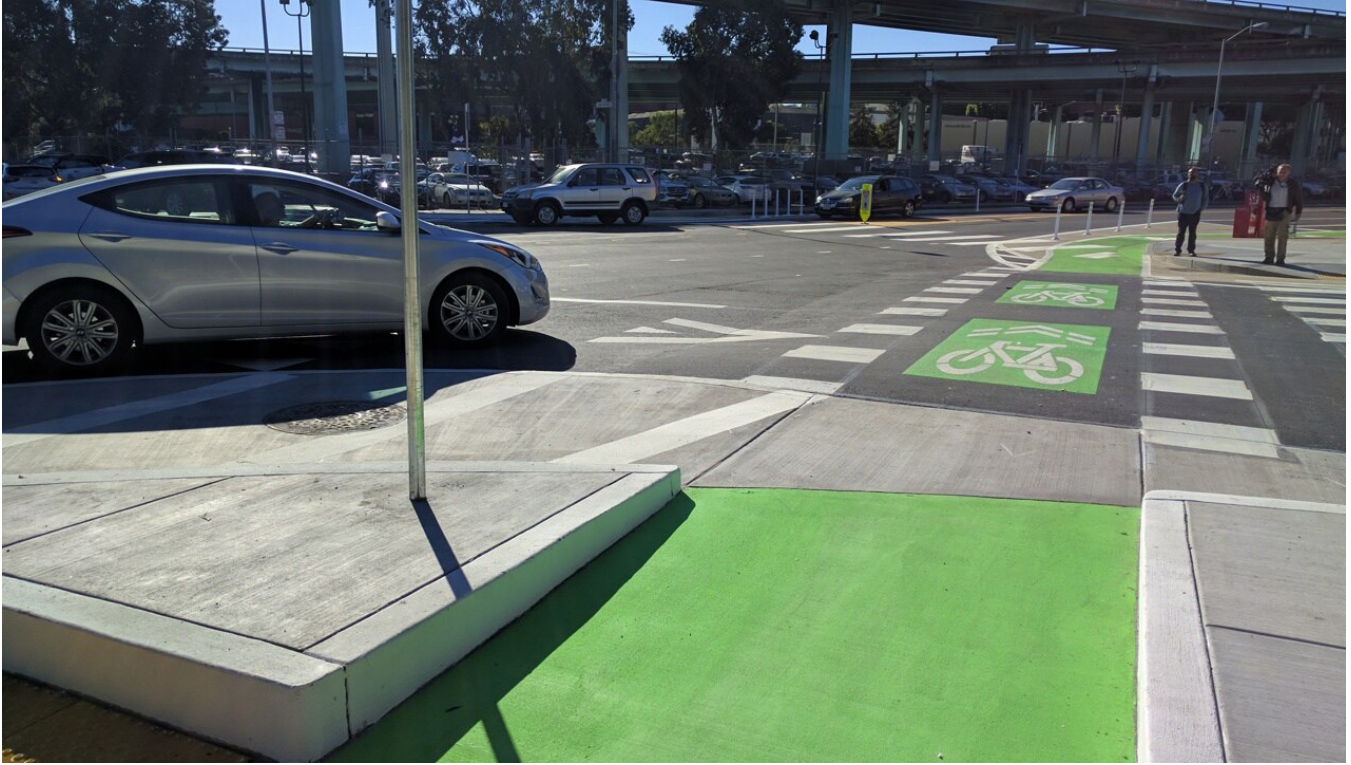
The 9th & Division Intersection has various corner designs featuring dual radius truck aprons created with striping and with raised concrete. Credit: StreetsblogSF. Source article
