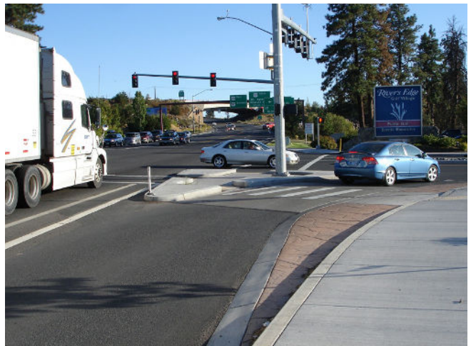
Right turn channel (Bend, OR)
