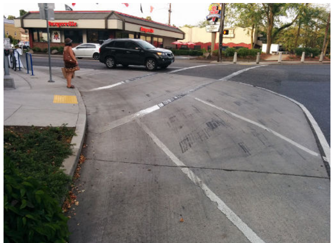
Signalized intersection (Portland, OR)
