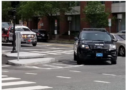
Gore striping/hatching (Cambridge, MA)
