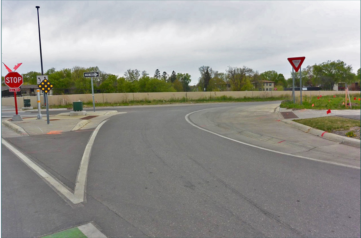
ABOVE: A road user's view of one of the right turn channels at the interchange with a traversable apron treatment.
