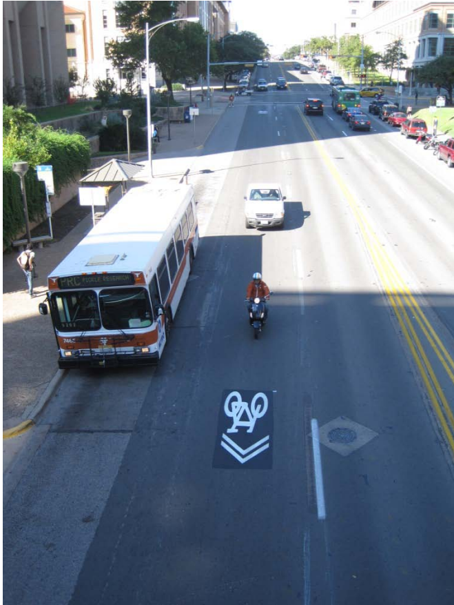
Figure B5. Central placement of sharrows on east-bound, downhill Dean Keeton St.
