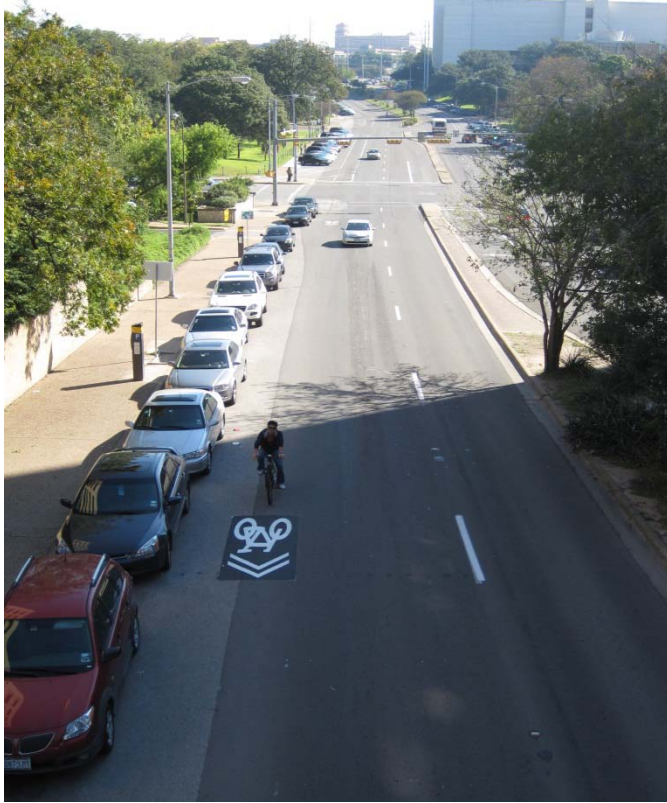
Figure B6. Curb-justified placement of sharrows on west-bound, uphill Dean Keeton St.
