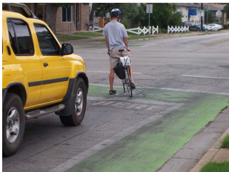
Figure B3. Poor quality of road lead to the deterioration of the thermoplastic bike boxes on Speedway Boulevard
