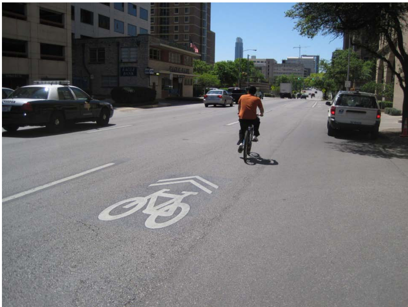
Figure B4. Central placement of sharrow resulted in thriving thermoplastic five months after installation.
