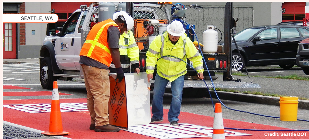
SDOT crews installing dashed bus lanes on Battery Street downtown.
