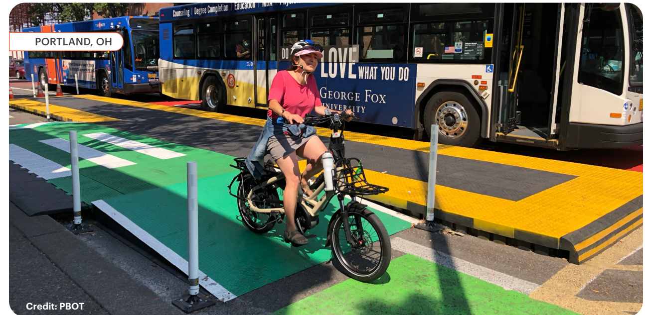
A Zicla bus boarding island and raised bikeway on SE Hawthorne street in Portland. 94
