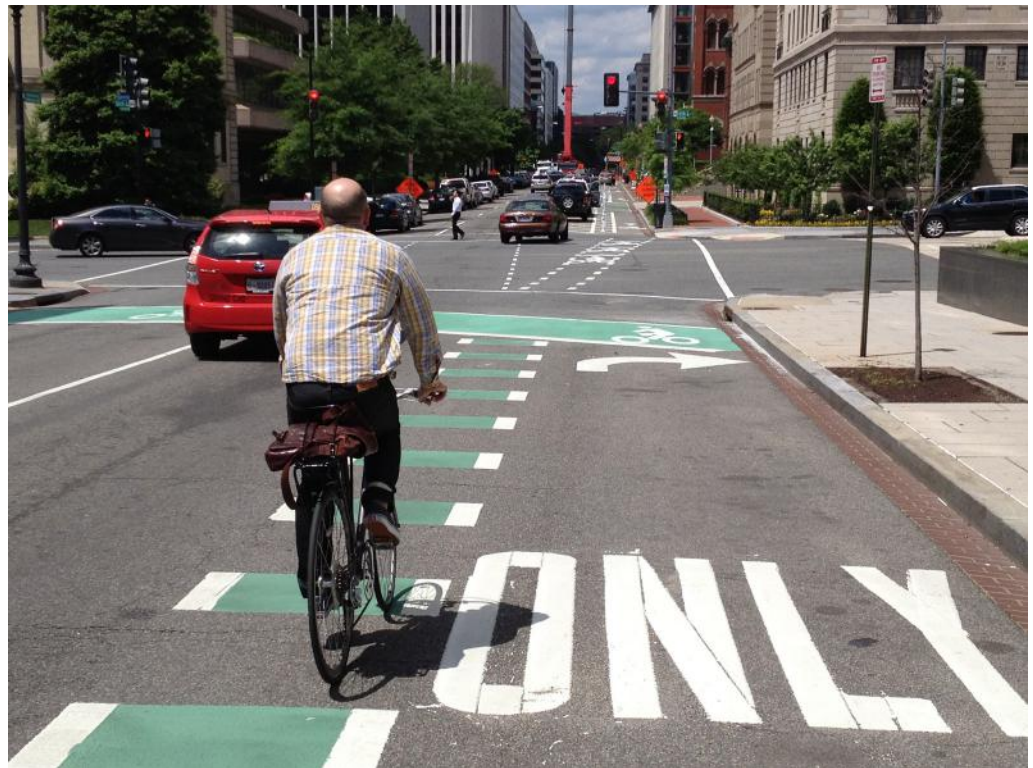
A cyclist approaches a bike box on M Street, Washington DC. Source: DDOT
