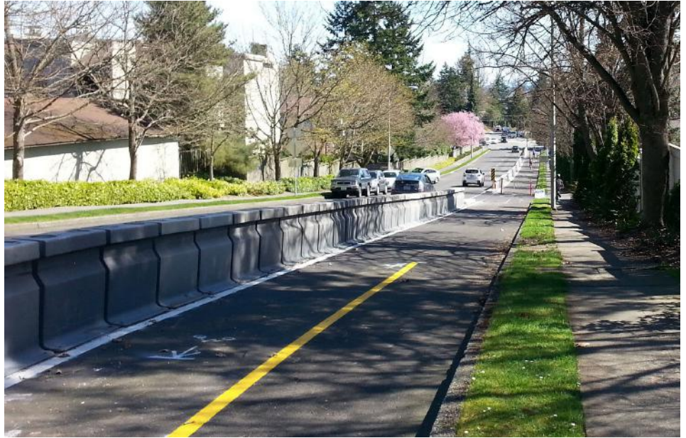
Seattle, WA. (Source: Seattle DOT)
