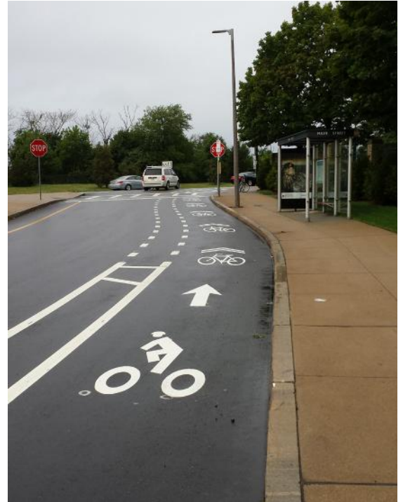
Shared bus stop/bike lane configuration in Boston, MA (Source: Conor Semler)
