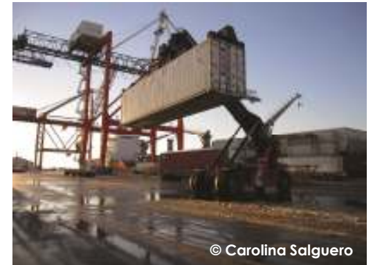
Red Hook Container Terminal, Brooklyn
