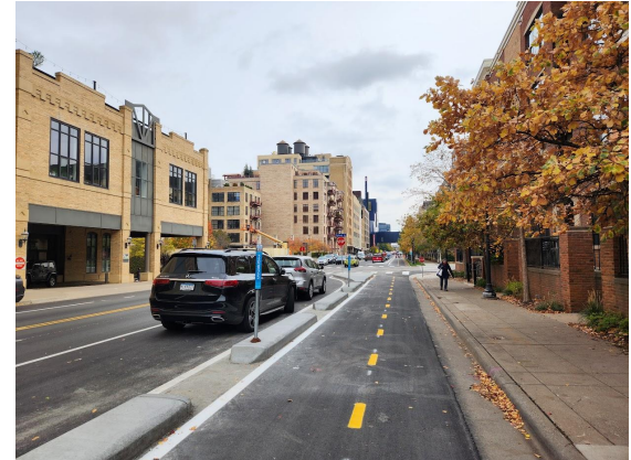
Buffer markings not required when physical separation occupies the "majority" of the buffer space
