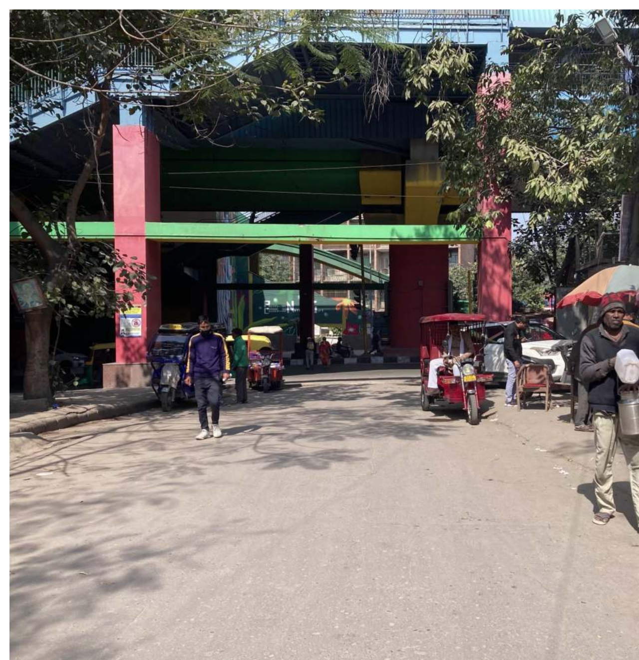
Connection 1: Rajendra Place Metro Station
