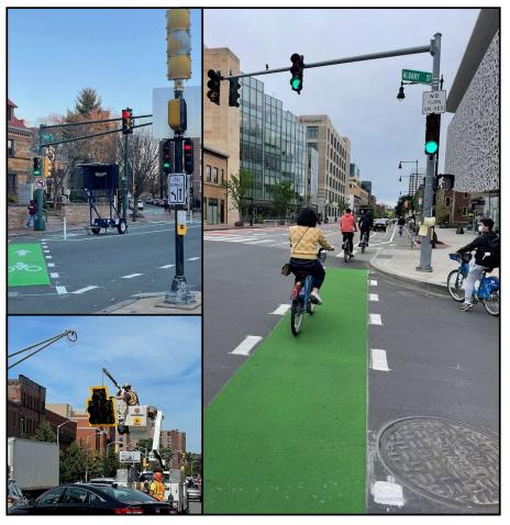
The City uses its on-call traffic signal contract to make spot improvements during quick-build projects. These include installation of bicycle signals (along with a leading bicycle interval) and flashing yellow arrows for vehicles. We have also been installing "No Turn on Red" signs at signalized intersections. Such upgrades align with the City's goals of moving people safely and encouraging new modes of transportation, thereby reducing dependence on single-occupancy vehicles.
