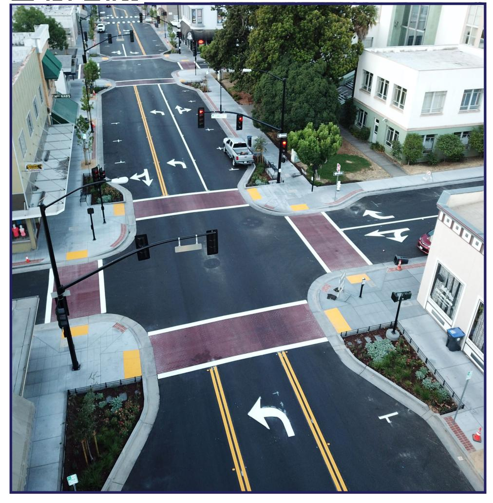
The project included "road diet" improvements to handle traffic volumes more efficiently with fewer lanes, enabling on-street parking, and safer pedestrian crossings with corner bulbouts. In addition to roadway reconstruction, the project also provided new ADA compliant sidewalks and pedestrian ramps, decorative brick highlights, modified traffic signals, street trees, decorative pedestrian streetlights, and a hybrid mid-block pedestrian crossing with a flashing beacon.
