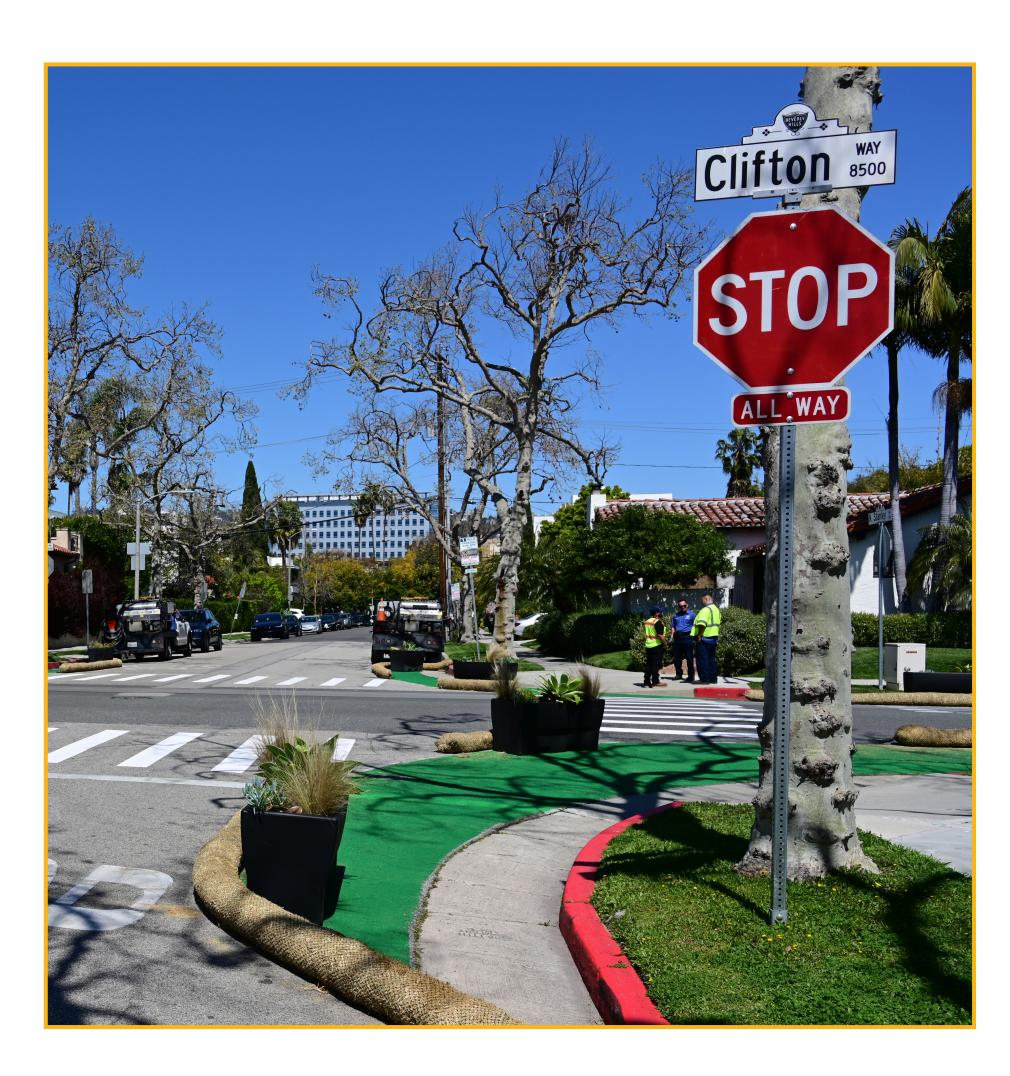
In March 2023, the City demonstrated temporary traffic calming devices that were determined feasible to install on either street. At two adjacent intersections, the community experienced temporary curb extensions with high visibility crosswalks and a traffic circle. The devices were made with tempera paint, straw waddles, traffic tape, planter boxes, potted plants, and a 48-inch boxed tree. After a 4-hour demonstration period, the City removed the temporary devices from the street.
