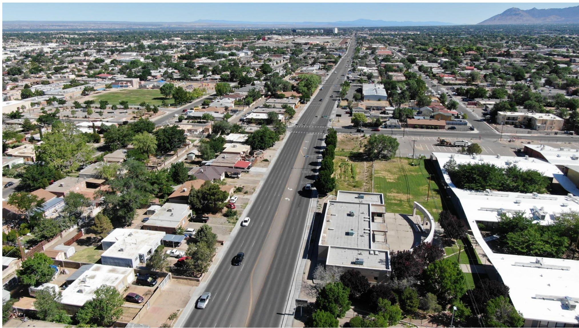
Louisiana Blvd looking north from Kathryn. The project corridor is approximately 1.2 miles.
