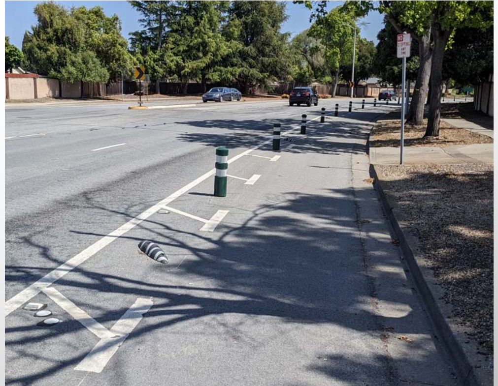
Combine K71 w/ Armadillo and Pavement Reflectors (after 6 months)
