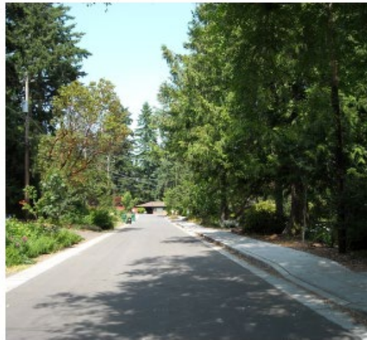
OD-2.3 Built example of reggraded street with concrete sidewalk and a consolidated bioswale on one side of the street
