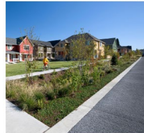
OD-1.2 Built example of porous asphalt in Seattle, Photo courtesy of Mithun
