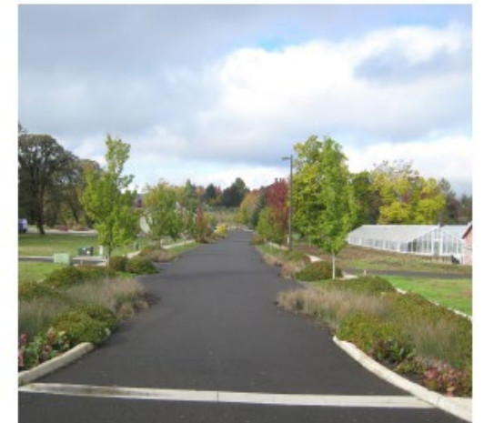
OD-1.2 Built example of porous asphalt in Pringle Creek; Photo courtesy Greenworks
