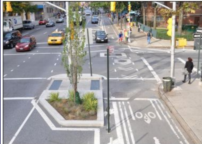
Left turn signal phase with bike signal on 9 th Avenue
