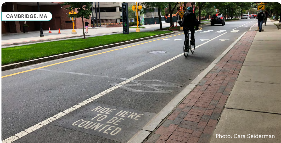
In-ground Inductive Loops installed in a bike lane.
