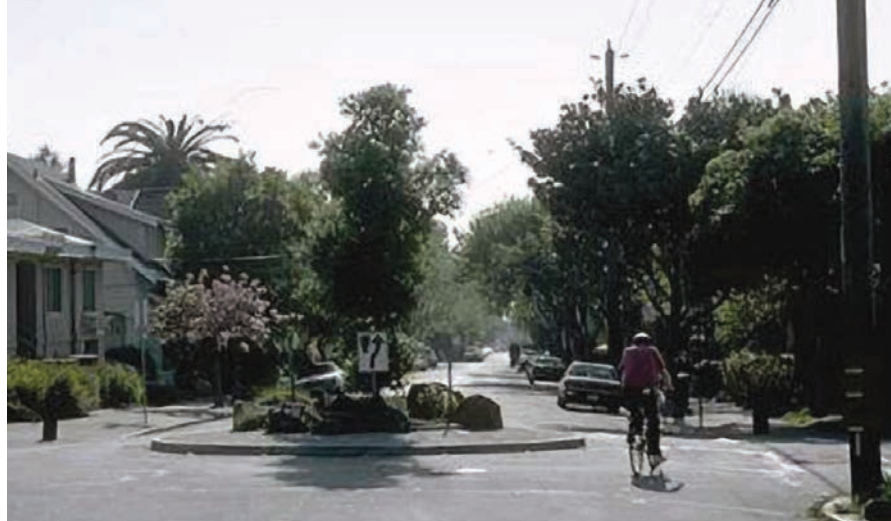
Neighborhood traffic circle with landscaping: Berkeley, California (Credit: John Allen) (Note: for illustrative purposes only)
