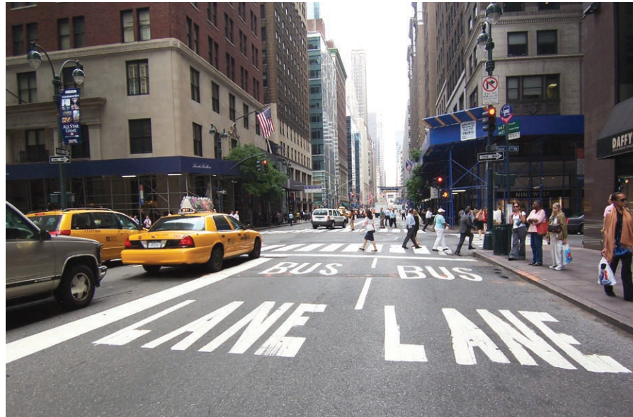
Curb-aligned double bus lane: Madison Avenue, Manhattan
