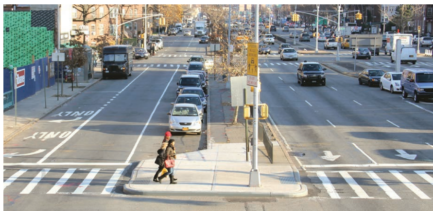
Wide roadways like Queens Boulevard can be mitigated with measures such as pedestrian facilities on medians: Queens
