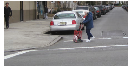
Curb extensions shorten crossing distances. This is especially important for vulnerable users: Fifth Avenue, Brooklyn
