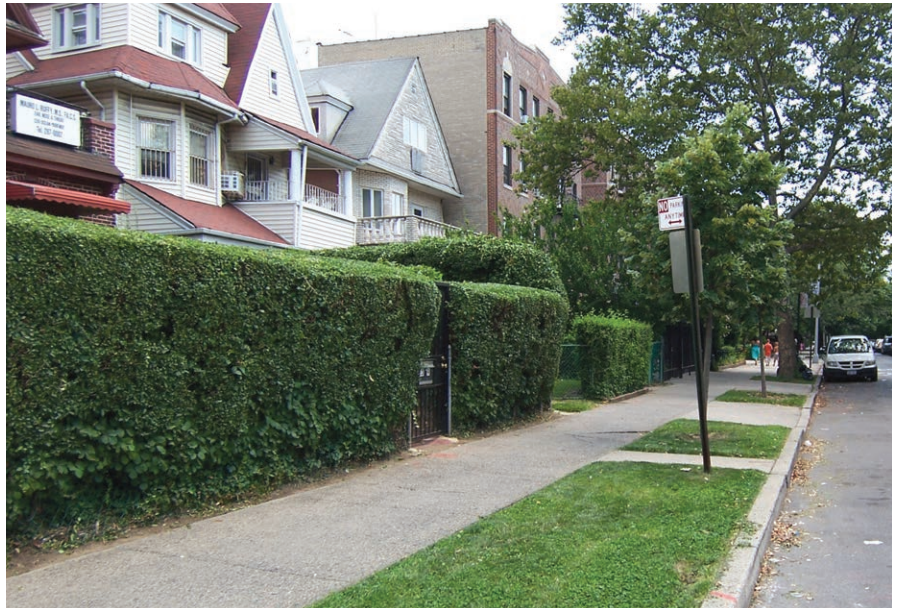
Ribbon sidewalk with lawn planting strip: Ocean Parkway at Avenue C, Brooklyn
