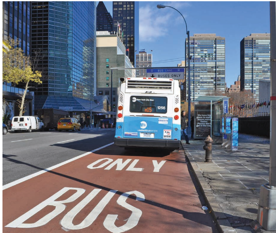
Red, curb-aligned, on-street busway with "soft separation" from traffic: First Avenue, Manhattan
