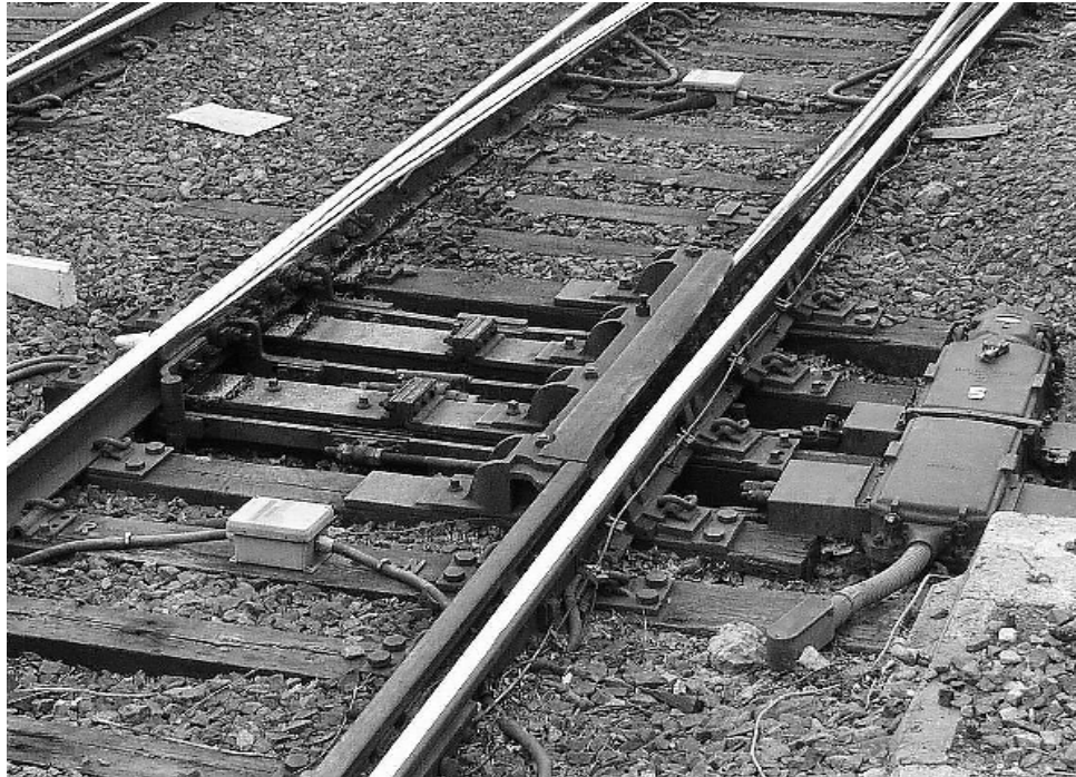
Figure 19. - Turnout with housed point.
