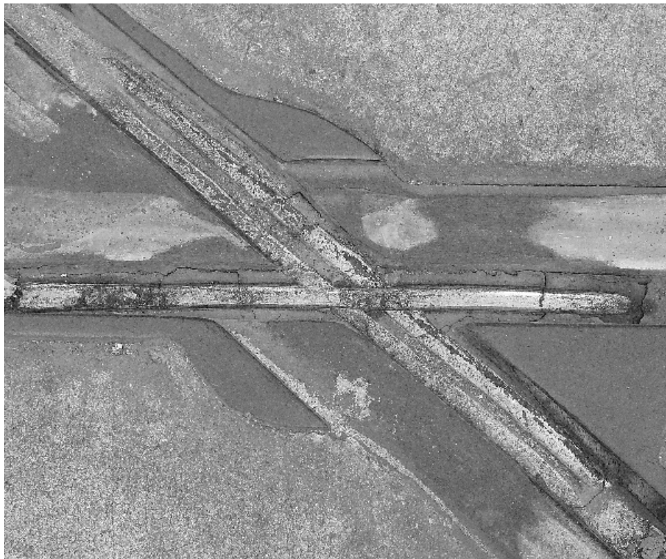
Figure 13. - Example of excessive gauge play.
