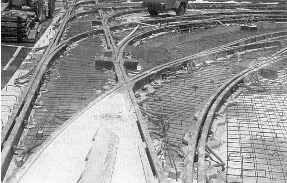
Figure 14. - Typical compact track fan at a storage facility but without gauging devices.
