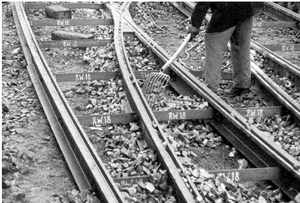
Figure 16. - Typical gauge bar application in a turnout.
