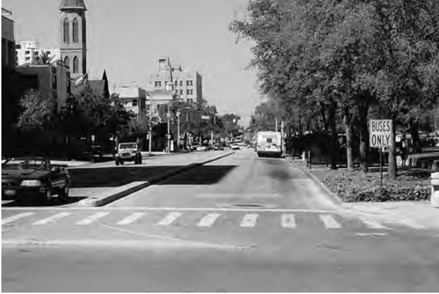
FIGURE 5 Contraflow bus lane on 4th Street, St. Petersburg, Florida (Source: Kittelson & Associates, Inc.).
