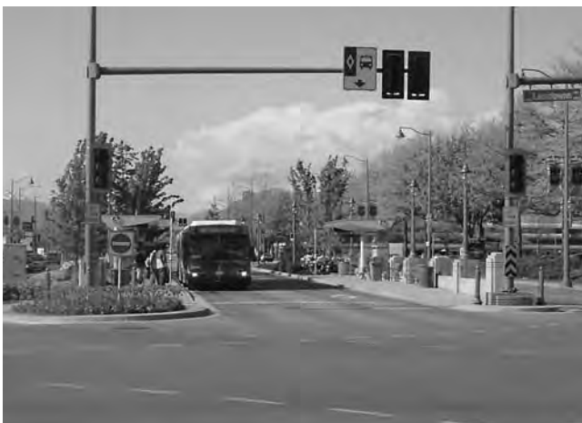
FIGURE 2 Former median bus transitway in Richmond, British Columbia (Source: Alan Danaher).
