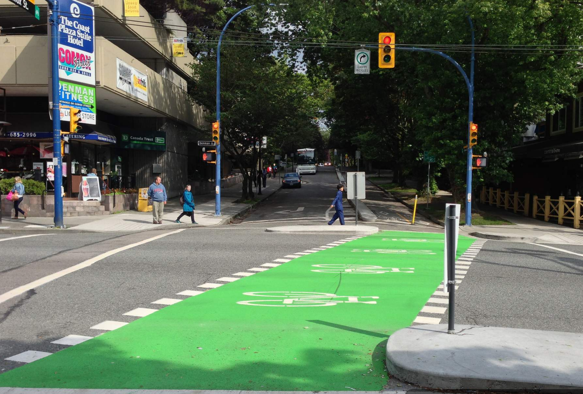
Comox Street and Denman Street
