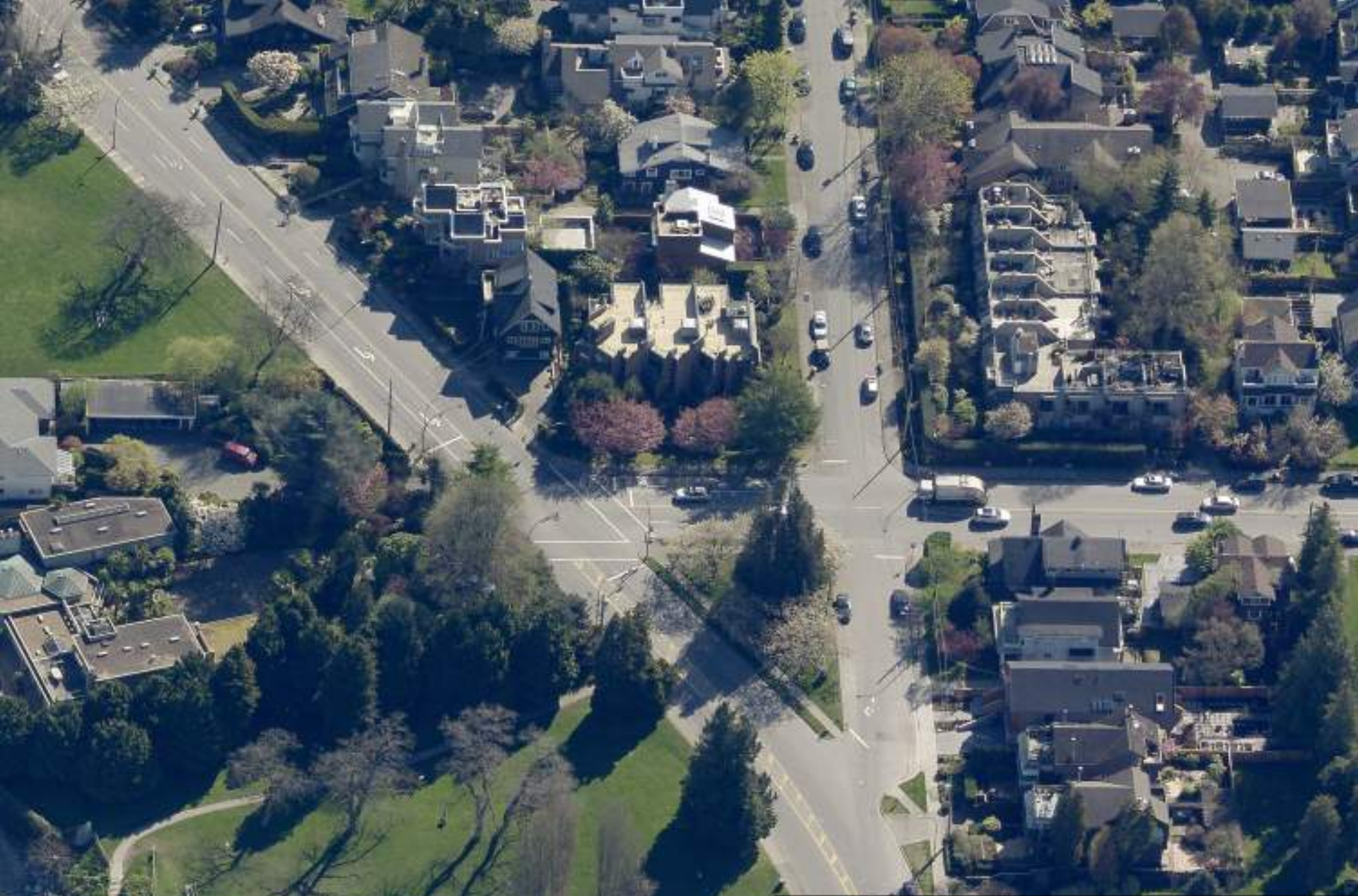
Macdonald and Point Grey Before Project
