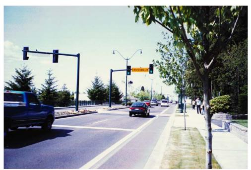
Figure 7-33. Example of a Midblock Signal in Washington.
