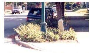
Figure 5-22. Example of a Curb Extension with Landscaping and a Bench.
