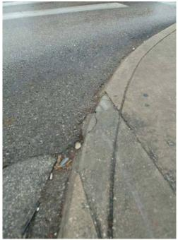
Figure 7-16. Uneven Pavement and Change in Level at Southeast Corner of Intersection.
