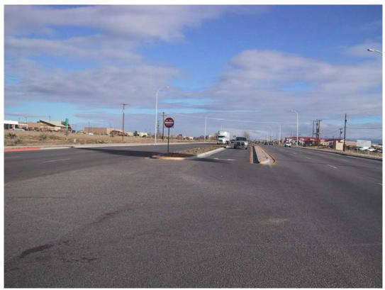
Figure 4-5. Example of an Offset Left-Turn Lane.
