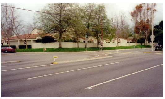
Figure 11-11. Channelized Median Opening to Restrict through Movements.
