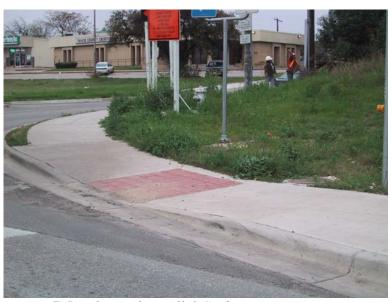
Figure 7-5. Photo of Parallel Curb Ramp.
