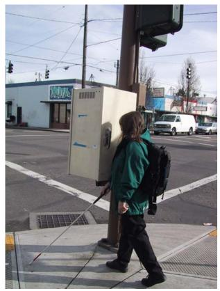
Figure 5-5. Protruding Controller Equipment.
