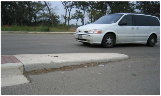
Figure 4-22. Ramped Down Median Nose.
