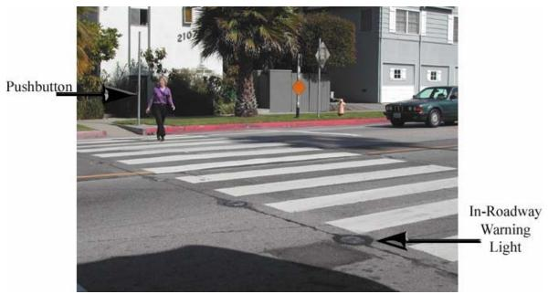
Figure 7-28. Example of In-Roadway Warning Lights.
