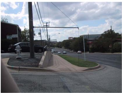
Figure 5-28. Guy Wire to Accommodate Pedestrian Movement.
