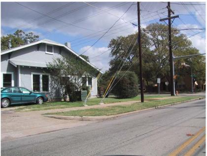
Figure 5-29. Guy Wire Parallel to Sidewalk.
