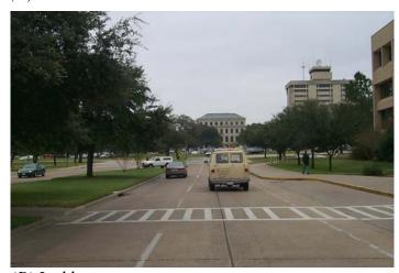
(B) Ladder Figure 7-11. Examples of Crosswalk Markings.
