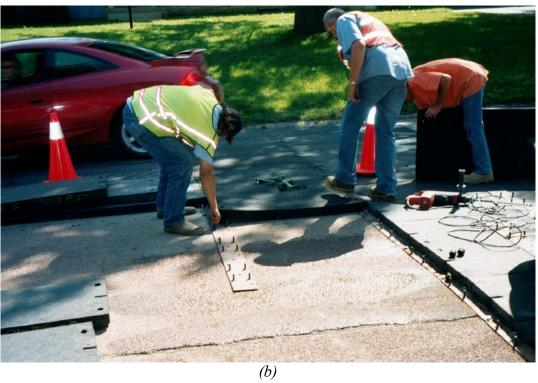
Figure B2. Temporary 30 mph Speed Table Installation.
