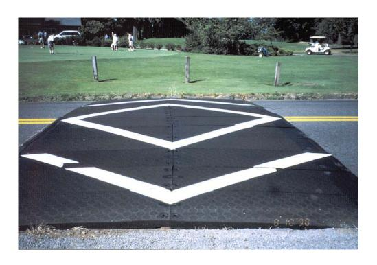
Figure 17. 14-Foot Temporary 25 mph Speed Hump (City of Portland, 2001)
