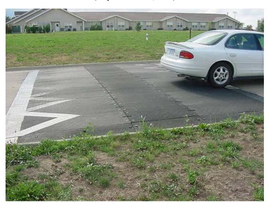
Figure 18. 18-Foot Temporary 30 mph Speed Table
