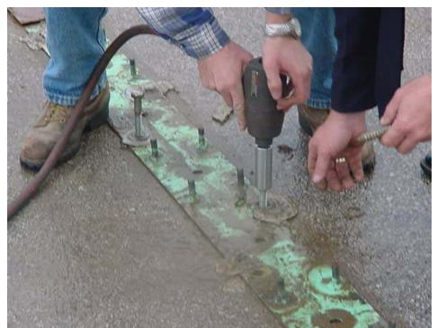
Figure B3. Lag Bolt and Anchor Plate Removal.
