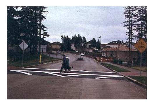
Figure 2. Typical Speed Table (Traffic Calming for Communities, 2001)
