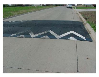
Figure 23. Pavement Markings on Speed Hump/Table
