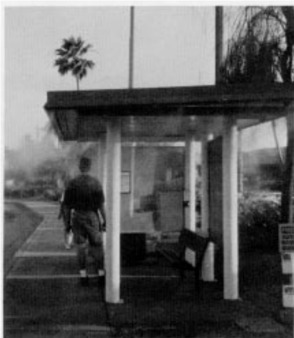
Figure E-27. Bus Stop Misting System.
