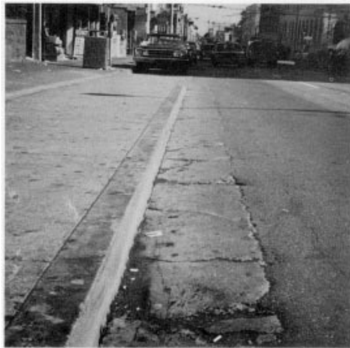
Figure D-6. Poor Pavement Condition at Bus Stop.
