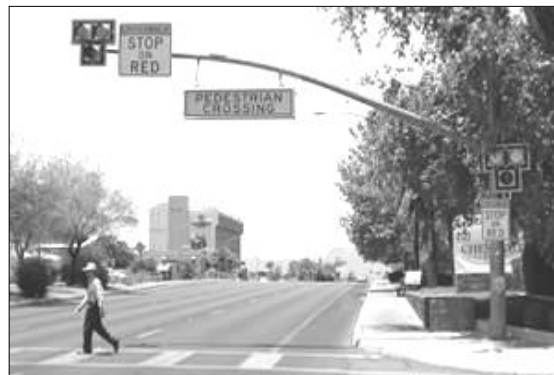
A HAWK signal, or H igh-intensity A ctivated C ross W alk, uses a signal with two red lights side-by-side, and a yellow light below; the signal is off when not in use and uses solid yellow, solid red, and flashing red to warn drivers.
