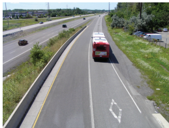
Figure 18 Direct-Access HOV On-Ramp
