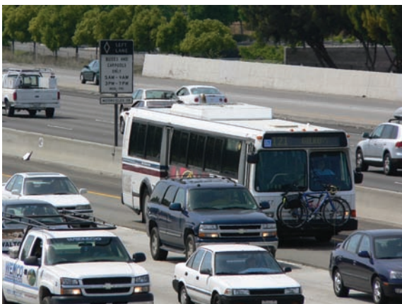
Figure 17 Median HOV Lane on Freeway with Striping
