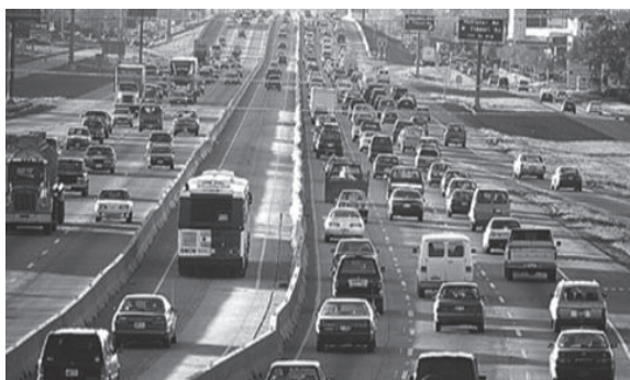
Figure 25 Median HOV Facility with Barrier (Houston)
