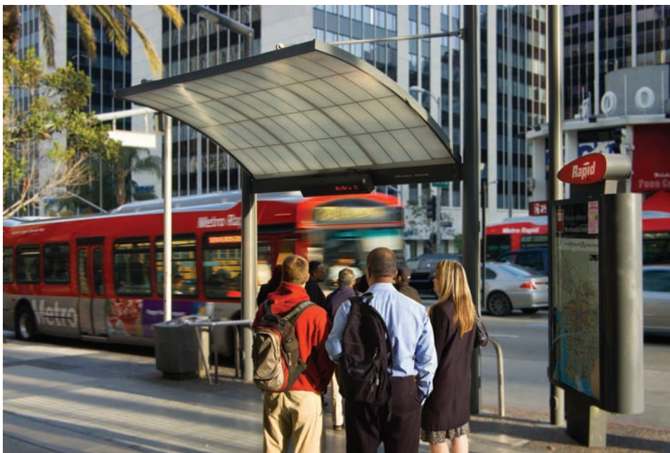
Figure 64 BRT 1 Type Curbside Station for BRT Using Mixed-flow Traffic Lanes (Wilshire Metro Rapid)
