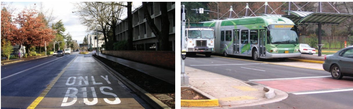
Figure 20 Designated Curbside Bus-Only Lane (Eugene)
