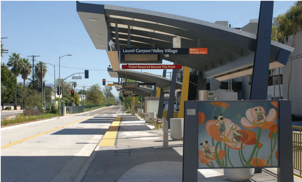
Figure 29 At-Grade Transitway (Los Angeles—Metro Orange Line)
