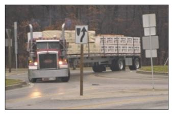
Good roundabout design makes accommodation for the appropriate design vehicle. For small roundabouts, this may require the use of an apron. *Lothian, MD*
