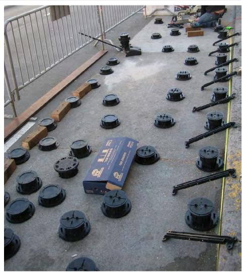
Figure 79. Bison pedestal system during installation, San Francisco, CA. Credit: SF Bicycle Coalition / sfbike.org
