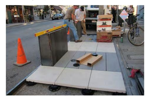
Figure 81. Pre-cast concrete pavers during installation, San Francisco, CA. Credit: Streetsblog SF
