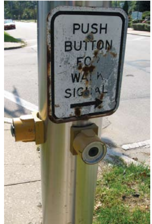
Signage that presents a shabby appearance may give the impression that the push button is old and will not work.
