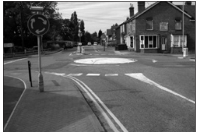
Figure 2. A mini-roundabout at a crossroad in the United Kingdom. This site features a 6-meter diameter domed roundabout; there have been two slight injury accidents in the 20 years since installation.
