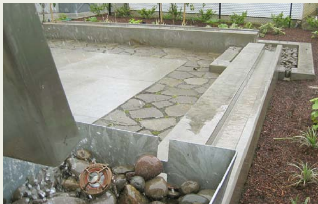
Local 49, Portland. Stormwater is conveyed from the rooftop by a decorative stainless steel metal scupper into the courtyard. Water flows from the scupper into a concrete runnel, detention basin and planters.
