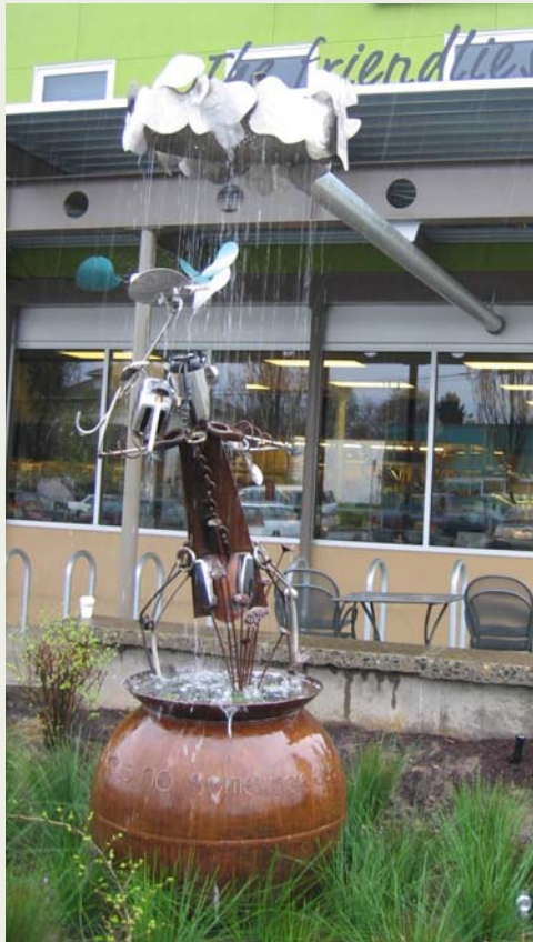
New Seasons, 20th and Division, Portland. A whimsical steel sculpture conveys stormwater from a grocery store rooftop into an infiltration planter.
