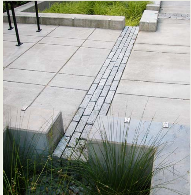
PSU Stephen Epler Hall. Stormwater from the impermeable plaza area is directed to bands of granite stone that are strategically placed at low drainage points to convey stormwater to a series of flow-through planters.
