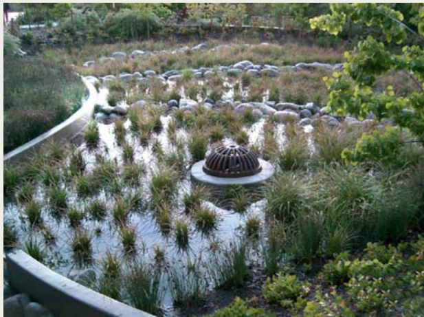
Glencoe Elementary School Rain Garden, Portland. Stormwater from neighboring streets is conveyed into an infiltration rain garden filled with native plants and rock berms that slow the flow of water. The rain garden is also a visual amenity and educational component for the elementary school (photo courtesy of 2008 Portland Stormwater Manual).
