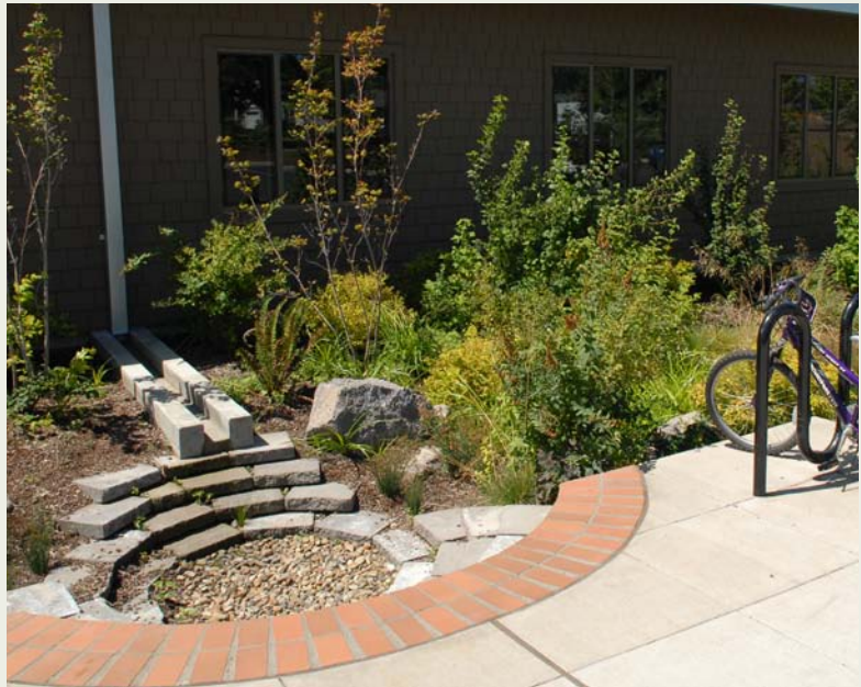
Estacada Library. Stormwater is conveyed from the rooftop to an infiltration basin. As the basin fills with water, it overflows into a connected series of swales and additional infiltration basins that convey stormwater around the library.
