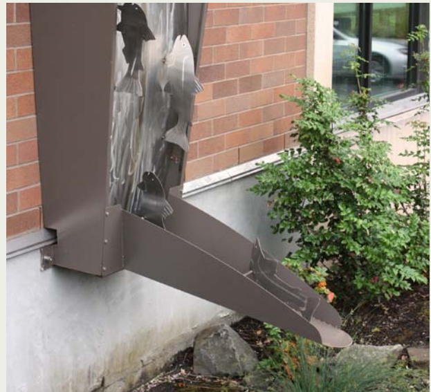
Glencoe Elementary School Rain Garden, Portland. Stormwater from neighboring streets is conveyed into an infiltration rain garden filled with native plants and rock berms that slow the flow of water. The rain garden is also a visual amenity and educational component for the elementary school (photo courtesy of 2008 Portland Stormwater Manual).
