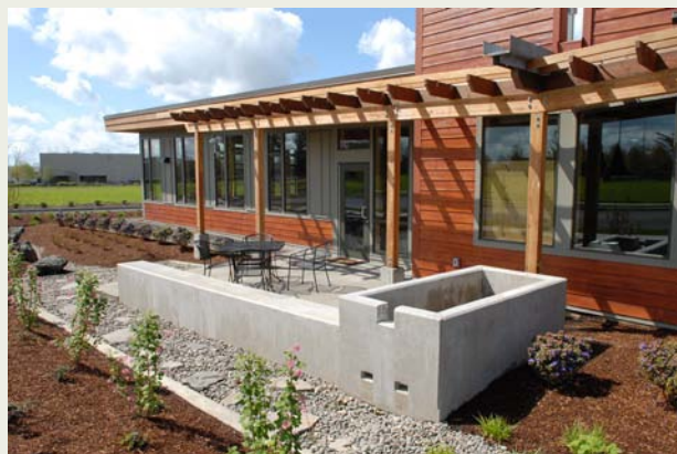
Team Estrogen Warehouse, Washington County. Stormwater from the warehouse roof is conveyed by a scupper into a concrete splash basin. The velocity of the water is slowed before the water flows into a vegetated swale.
