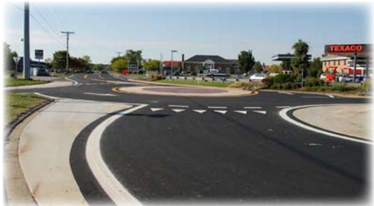
Figure 8: Example Mini-Roundabout
