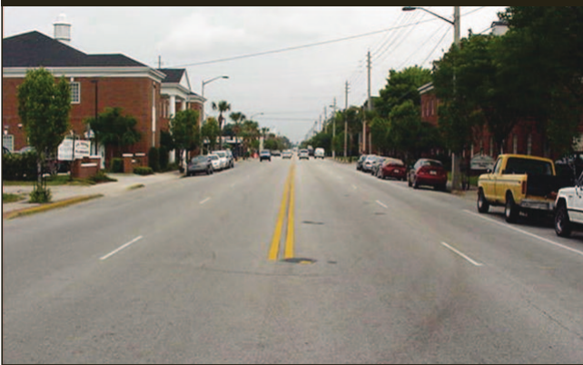
Figure 1. Photo. Four-lane configuration before road diet.
