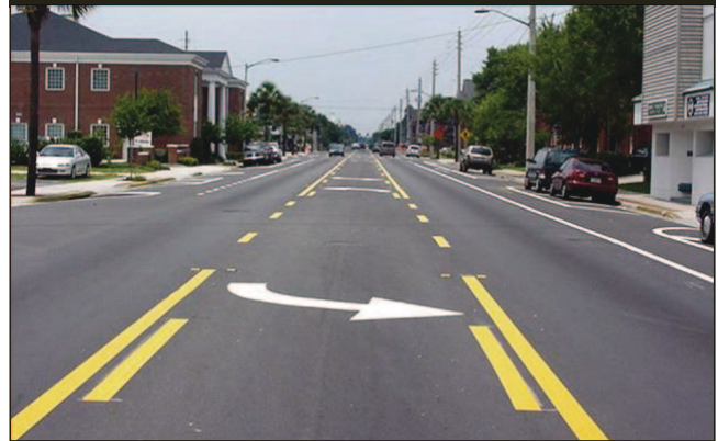
Figure 2. Photo. Three-lane configuration after road diet.
