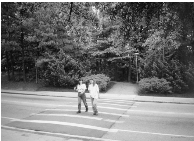
FIGURE 2 Two pedestrians using raised crosswalk.
