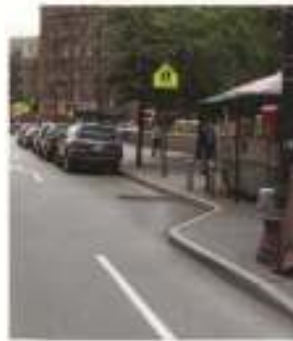
Curb Extension, Seventh Avenue, Manhattan
