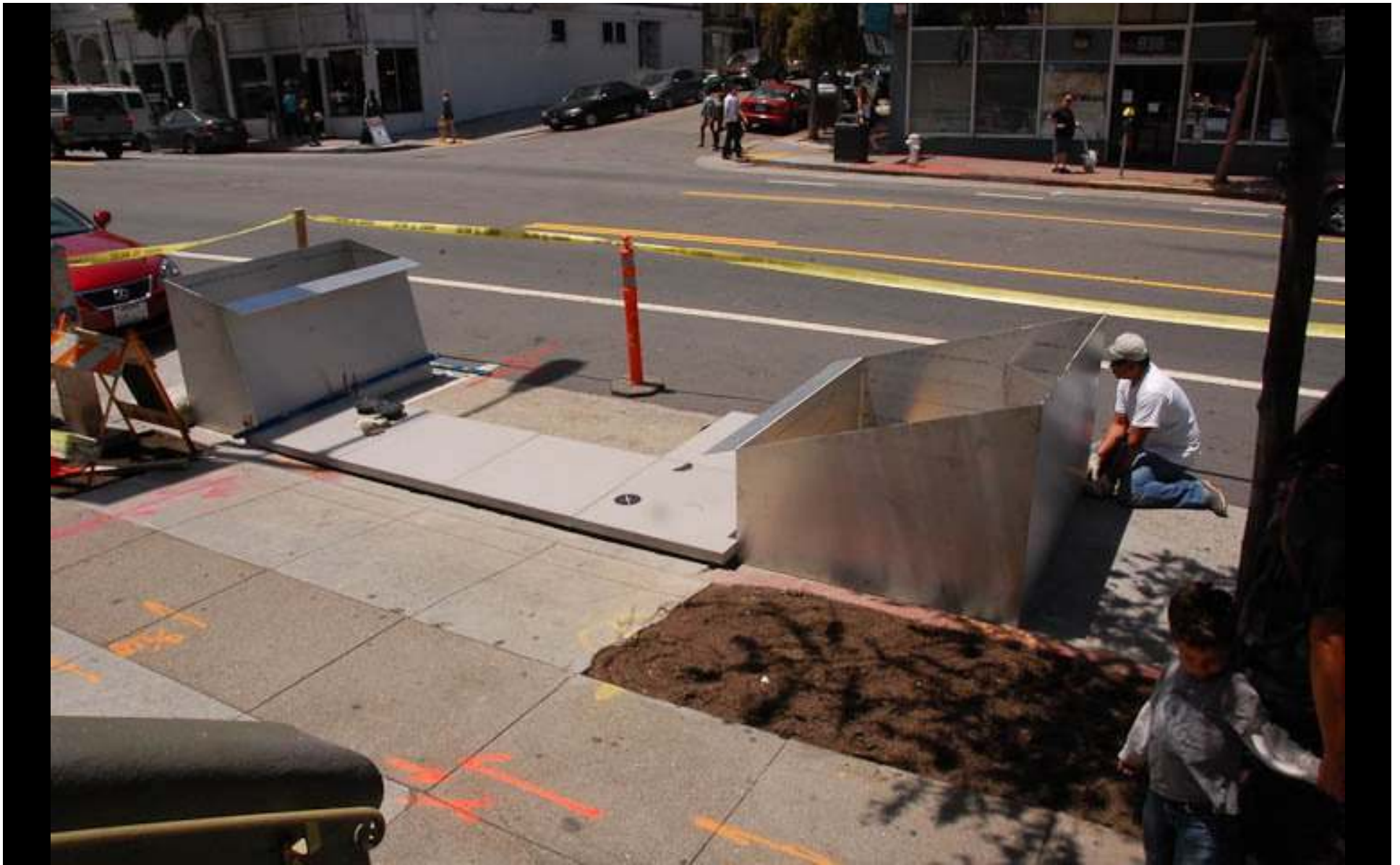
Materials pre-assembled off-site for quick installation time
