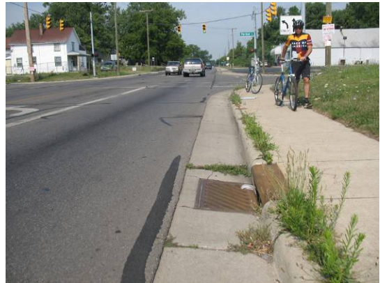
Roadway resurfacing should ensure that the transition between the asphalt and the gutter pan is flush, with no lip.
