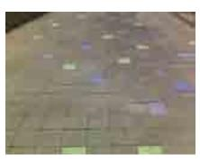
Concrete pavers with exposed blue and green glass aggregate (shown interspersed with black asphalt pavers): Hudson River Park, Manhattan
