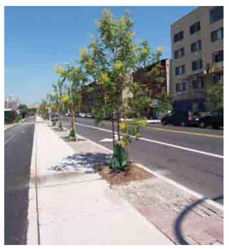
Connected tree pits with permeable paver-covered trench: Columbia Street, Brooklyn
