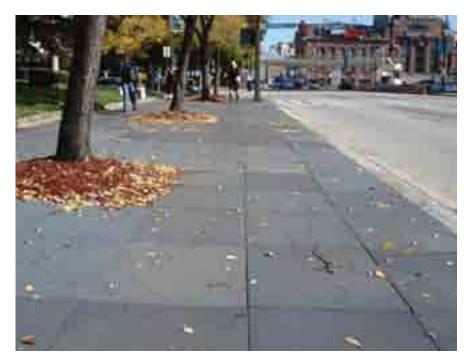
Rubber sidewalk pavers (credit: Rubbersidewalks®)
