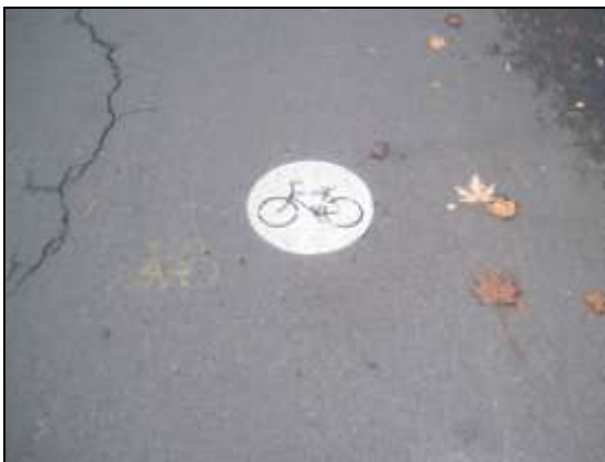
Figure 5 Bicycle boulevard pavement markings on SE Salmon Street.
