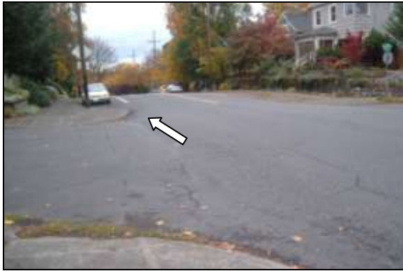
Figure 3 Curb extensions help reduce cross-traffic speed on SE 30th Ave.
