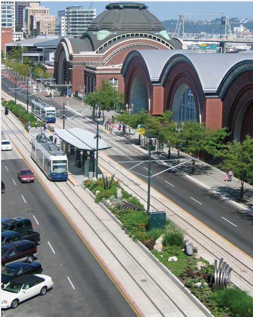
Tacoma Link Light Rail
