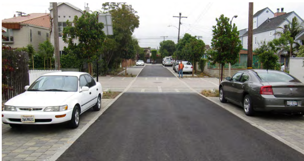
Longfellow Street, a Living Street , in Santa Monica, designed by Nelson\Nygaard.
