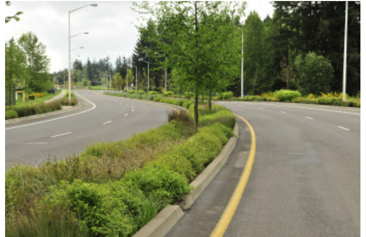
Tuluatin, OR – 124th Avenue Green Street Median
