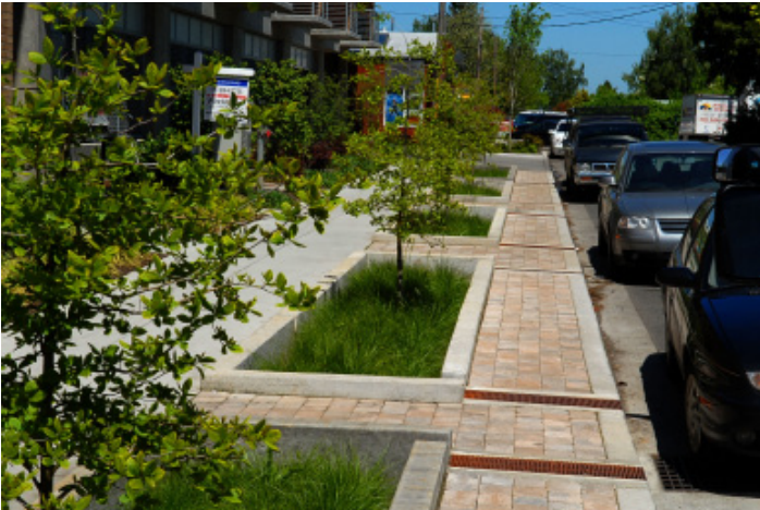
Beaumont Village Lofts Stormwater Planters
