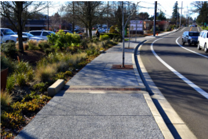
Warner Milne Pervious Sidewalk
