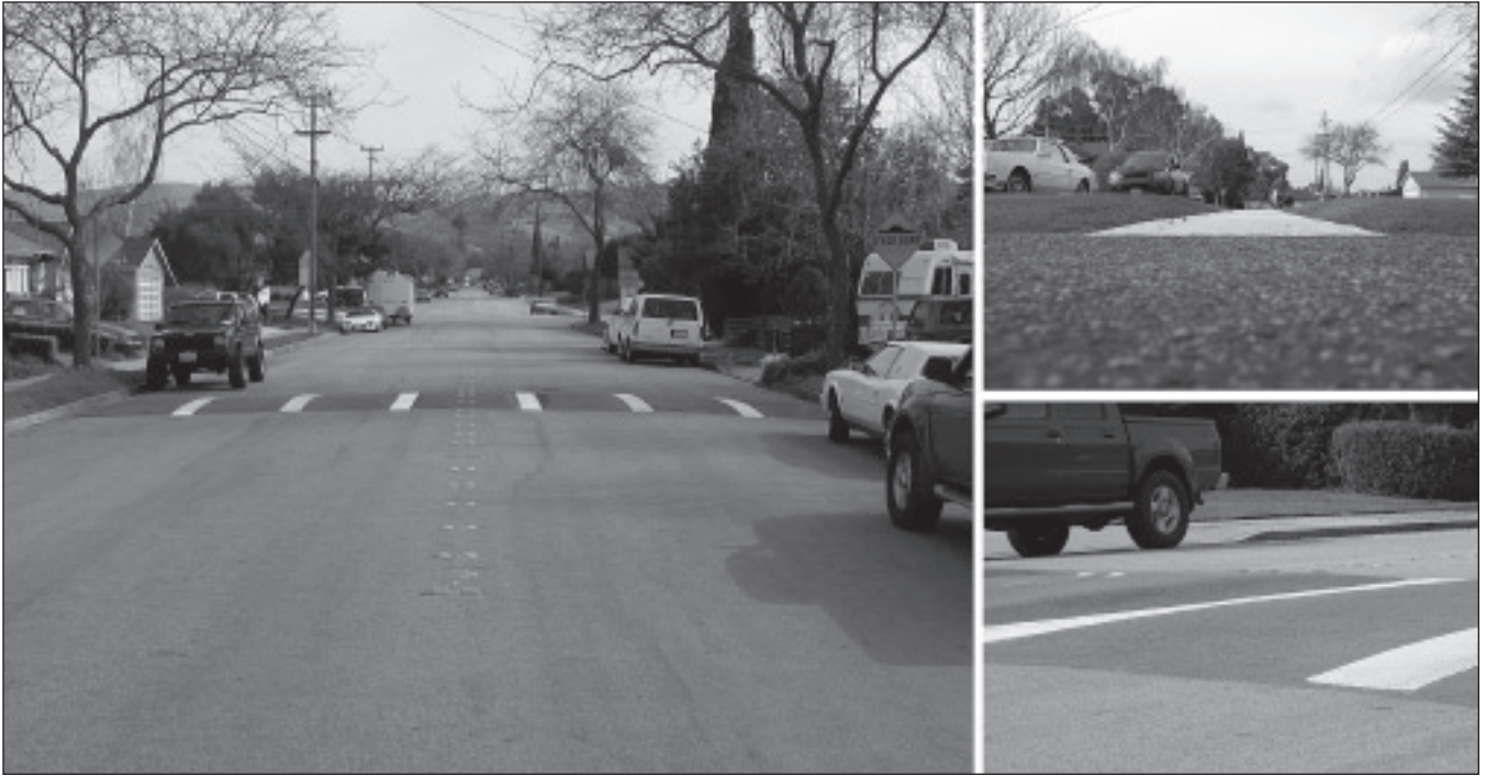
Figure 4. Speed lumps striped to appear as a speed hump in Fremont, California.
