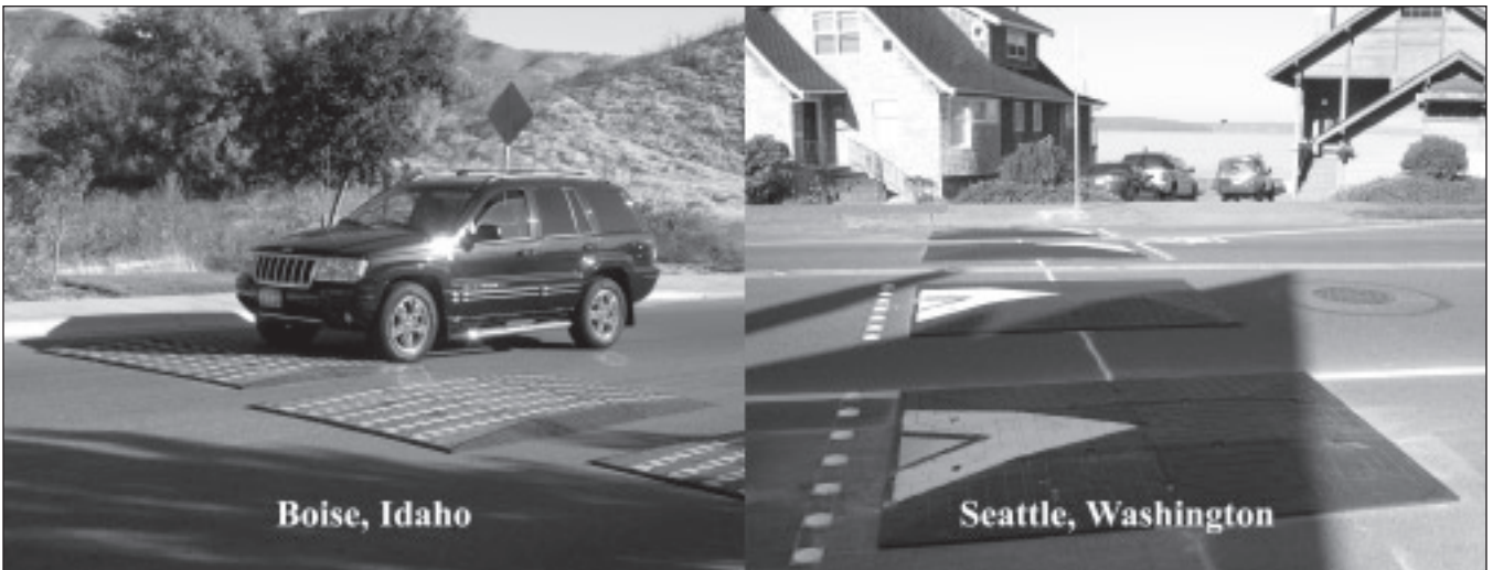
Figure 2. Common prefabricated rubber speed lumps.
