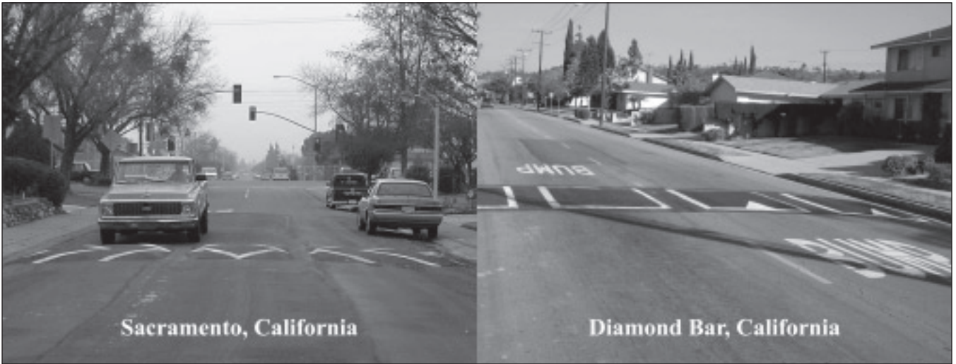
Figure 1. Typical asphalt speed lumps.
