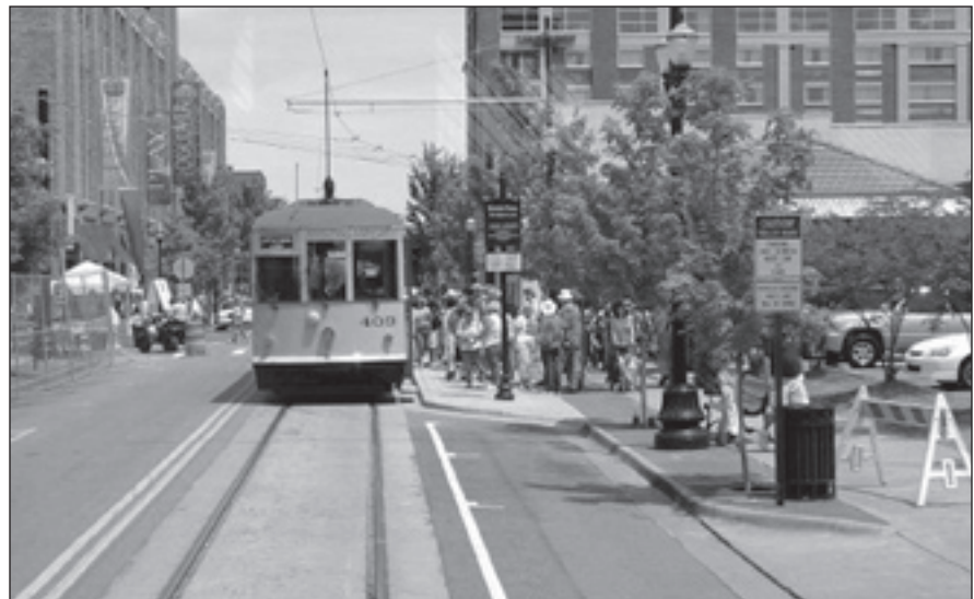
Figure 2. Curbside bulb-out for platform—Little Rock, Arkansas, USA.
