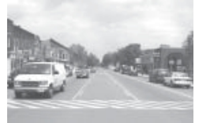
Where traffic volume, speed or other conditions warrant, four-lane highways can be reduced to two-lane designs using raised medians or turning medians.
