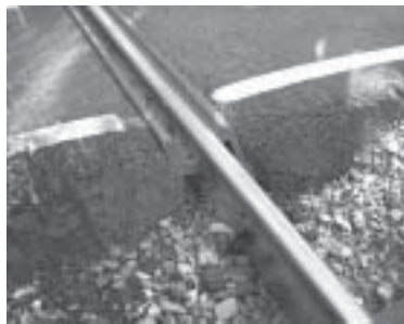
Rubberized flangeway fillers can smooth railroad track crossings for bicyclists.
