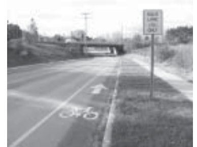
Bicycle lanes, designated by signs, stripes and symbols, are intended for the preferential or exclusive use of bicyclists.
