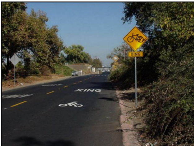
Advance marking and signage for a mid-block bike crossing in Sacramento, California.
