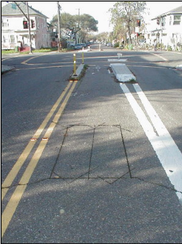
Advanced inductive loop traffic signal detector on Channing Street at Martin Luther King, Jr. Way in Berkeley, California.
