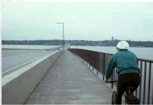
Floating Bridge, Seattle, Washington
