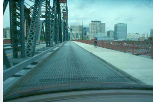
Bridge with Metal Grate Deck, Portland Oregon
