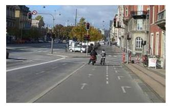
Figure 13. Straight and right turn (extended cycle stacking lane) at intersection, Copenhagen
