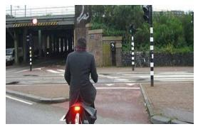
Figure 20. Cycle track crossing streetcar tracks, with pavement yield markings
